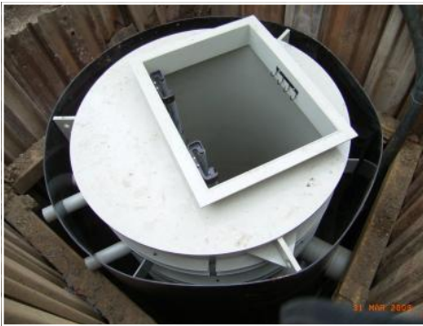
Prefabricated Pumping Station with optional shuttering to accept concrete pour
