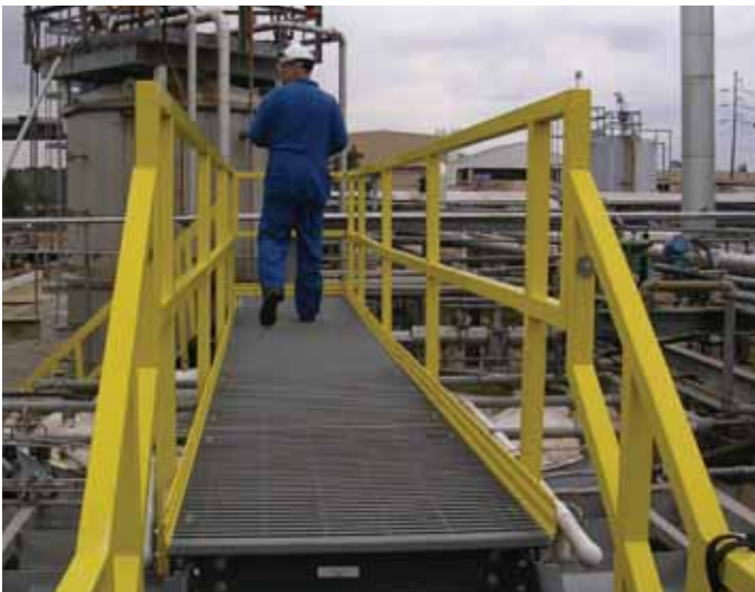
SAFRAIL™ and DURAGRID® pultruded grating were fabricated to make access platforms over waste water recycling tanks. The previous steel structure corroded, and was unsafe.
