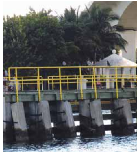
In 2002, Fort Lauderdale, FL received the very first installation of Strongwell's round SAFRIL™ on the 17th Street Bridge's fenders. Inspection in 2010 (shown here) revealed that 8 years of exposure to the Florida sun and the Atlantic Ocean have resulted in no corrosion related issues.
