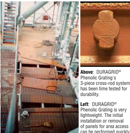
DURAGRID® Phenolic Grating's unique construction allows for many penetrations to be cut without adding additional supports.
