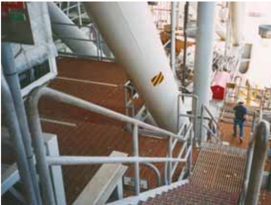
DURAGRID® Phenolic Grating has been used to reduce weight and maintenance on offshore oil production platforms for more than a decade.
