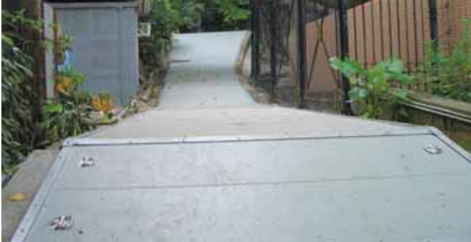
SAFPLANK® panels are used as air-tight drainage covers in a residential area of Hong Kong for odor control. The lightweight panels provide a safe walking surface and also allows easy access below the covers.
