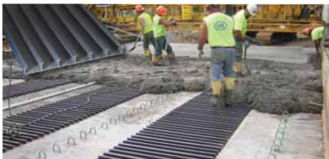
SAFPLANK®, when turned upside down, serves as an excellent concrete forming system in applications where corrosion and weight are construction concerns.
