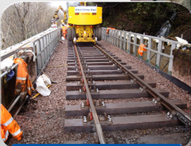
FRP Bridge Deck Complete Installation
