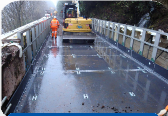
Railway Bridge Deck
