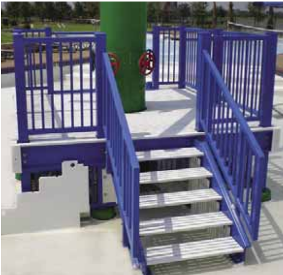
Above: A fiberglass waterpark platform in Cypress, Texas was fabricated using EXTREN® structural shapes, DURAGRID® pultruded grating and STRONGRAIL™ fiberglass architectural handrail.
