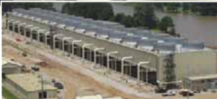
Above, Right: Fiberglass has become the material of choice in the cooling tower industry because of the many advantages it has over wood.
