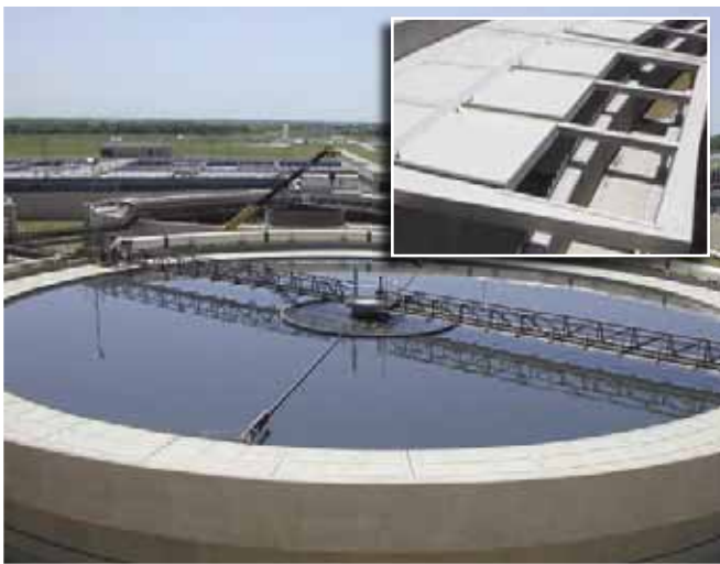
Above: FRP odor control covers around the perimeter of wastewater treatment tanks in Grand Prairie, Texas, were fabricated using COMPOSOLITE® and DURASHIELD® structural panels, EXTREN® and several custom shapes.
