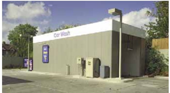
Above: This car wash is constructed using COMPOSOLITE® 3-way connectors, toggles and panels. Low maintenance, ease of construction and an attractive appearance were the primary benefits to the customer.
