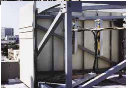
Left: EXTREN® fiberglass plate and structural shapes were used for cellular antenna enclosures. The enclosures were designed to match the style and appearance of the Santa Ana Historical building.
