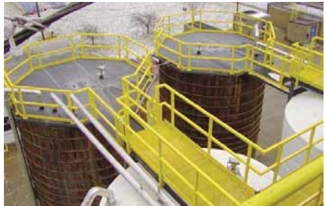
Above: These tanks are surrounded by SAFRAIL™ and DURADEK® walkways and covered with COMPOSOLITE® covers for odor control.
