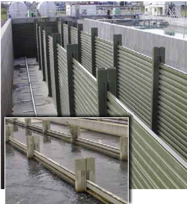
Above: Lightweight, corrosion resistant 24" fiberglass I-beams span 45' to bridge clarifiers at a wastewater treatment plant in Las Rusias, Texas.
