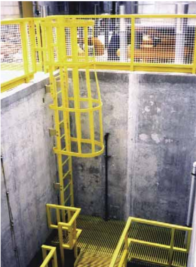
Above: Fiberglass access ladders and walkways used throughout the service areas of Sea World in Orlando, Florida, resist saltwater corrosion and reduce maintenance costs.
