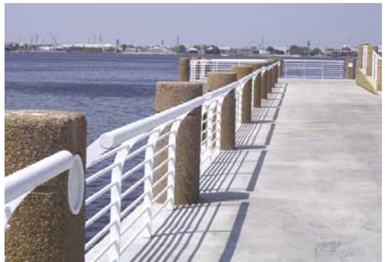
Above: A custom fiberglass architectural handrail system is the ideal solution for corrosive coastal environments like this theme park pier in Galveston, Texas.
