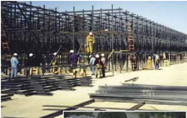
Above, Right: Fiberglass has become the material of choice in the cooling tower industry because of the many advantages it has over wood.
