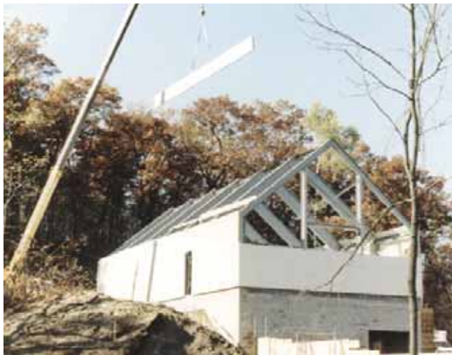
Above: This all-fiberglass facility for Amador Corp. assures RFI/EMI compliance in testing computers as well as other manufactured equipment.
