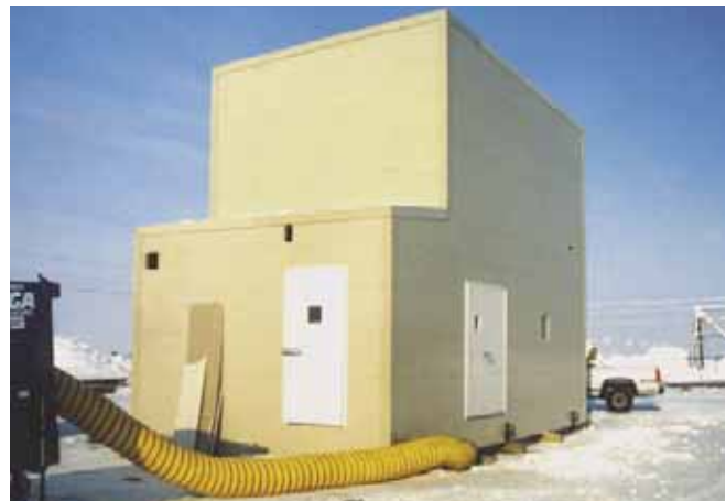
Above: DURASHIELD® foam core building panels and EXTREN® Series 525 fiberglass shapes were used to fabricate this fiberglass building in Alaska. DURASHIELD® was selected for this project for its durability, light weight and thermal properties.
