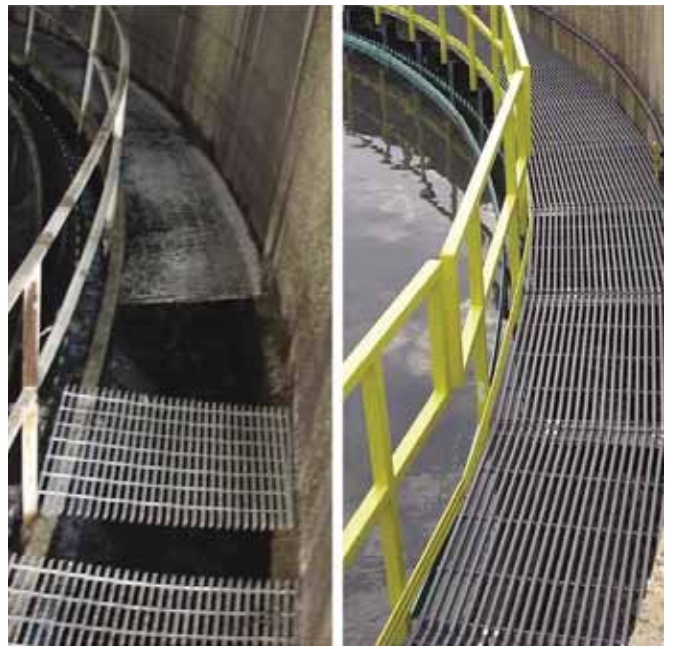
Above: Low maintenance fiberglass grating, ladders and handrail replaced steel to provide trouble-free operations for a wastewater treatment clarifier in Albert Lea, Minnesota.
