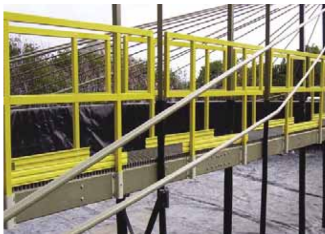
Above: This corrosion-resistant fiberglass walk-over bridge platform allows the Oceanic Marine Institute in Hawaii to monitor large batches of shrimp under research.
