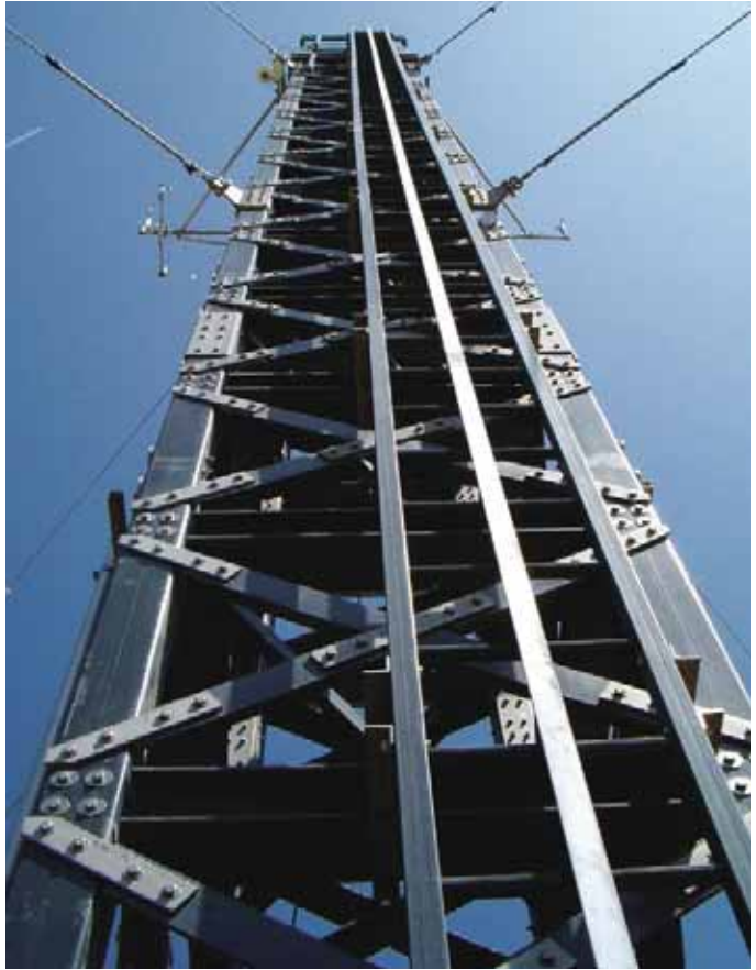
Above: A 62" tall weather tower at Vandenberg Air Force Base near Santa Barbara, California, is composed of EXTREN® structural shapes, ladders and DURADEK® pultruded grating.
