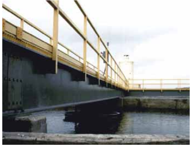
Above: Lightweight, corrosion resistant 24" fiberglass I-beams span 45' to bridge clarifiers at a wastewater treatment plant in Las Rusias, Texas.
