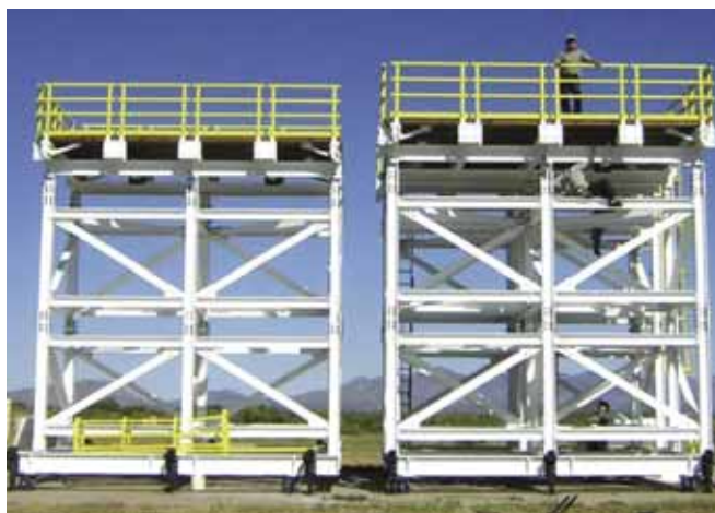
Above: A pair of platforms constructed using Strongwell's FRP products is used by the U.S. Army to help test the radar systems of its helicopters, troop
