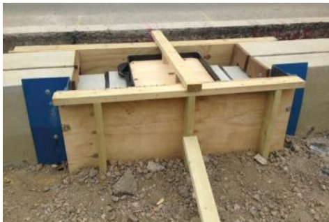
Interconnecting slot drain former with timber shuttering
