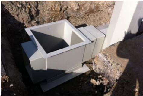
Thermoplastic outfall chamber during installation on the M3, UK
