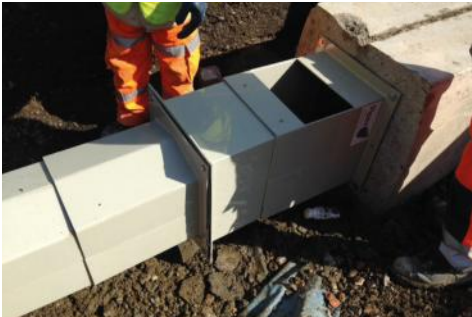
Thermoplastic access point fitting during on-site installation, UK
