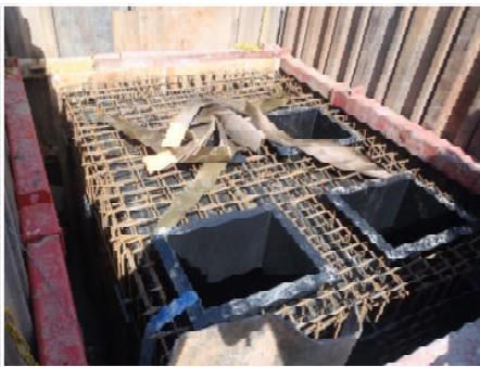
Optional reinforced top formwork with access turrets
