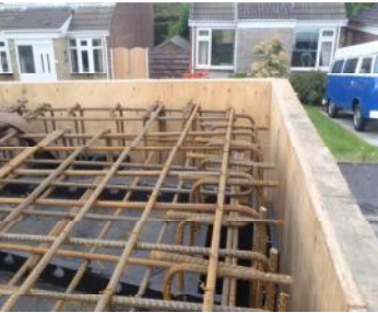
Fast track installation minimising disruption to residents
