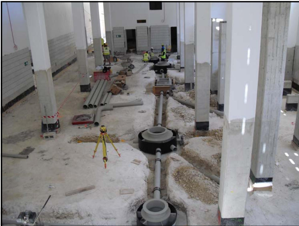
(Pipex px ® manholes & associated pipe work during the installation process and concrete surround)
