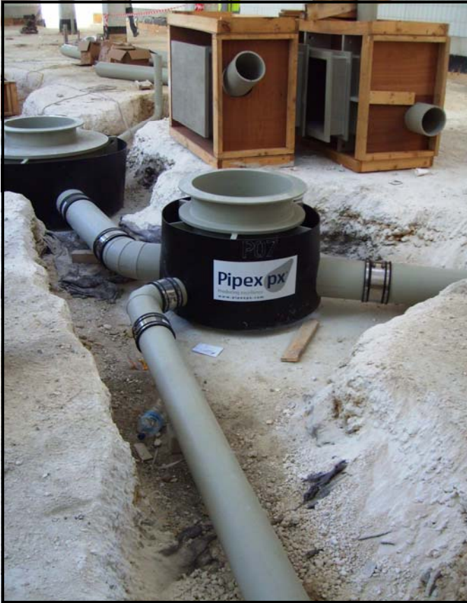
(Pipex px ® manholes & associated pipe work during the installation process and concrete surround)
