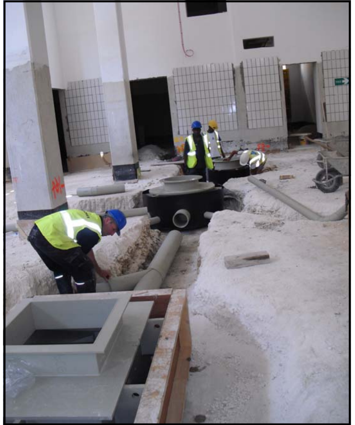
(Pipex px ® manholes & associated pipe work during the installation process and concrete surround)
